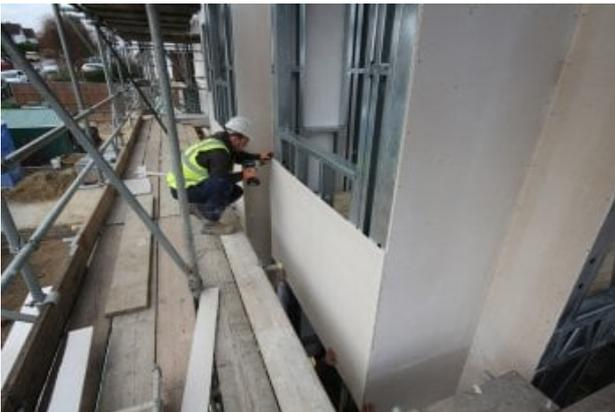
While in respect to this project, the UniFrame system includes diagonal ties which are tensioned on site, Magply is often used by timber frame manufacturers to take the racking loads for their buildings as well as to provide fire protection in close proximity to other properties.
