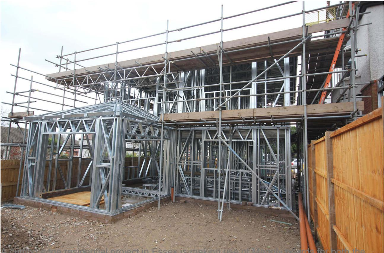
A cutting edge residential project in Essex is making use of Magply boards for both the internal lining and exterior cladding treatment to an innovative lightweight steel framing system, demonstrating the widely specified fire resistant product's multiple attributes.
