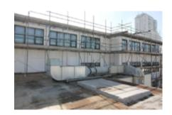
This is a very large and quite complex building, with some parts being very exposed and high. Our operatives started by screw fixing the Magply boards over battens secured to the original external walls and we are now applying the K-Rend in a process which will take a total of just three weeks, despite the weather having been poor early on.
