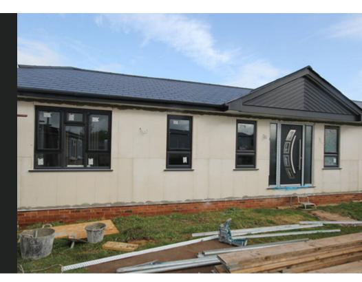
High performance Magply boards have been selected as the substrate for a bright white silicone render system, used as a striking finish to a single-storey, modularised domestic property on a green-field site in Kent.
