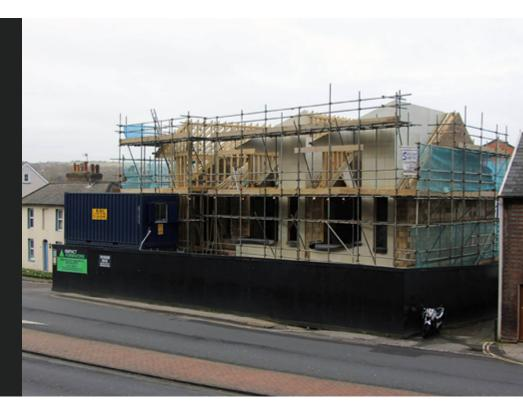
A development of five stylish townhouses in East Sussex three of which feature the traditional finish of slate hanging, fixed across Magply boards with horizontal battens, providing a substrate offering excellent weathering and fire resistance, as well as a secure fix.
