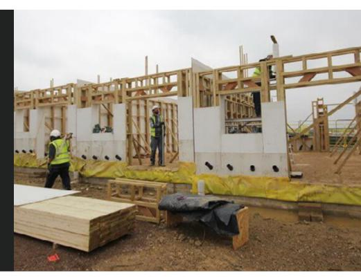
UK based PassivHaus specialist is employing Magply modified MgO boards as part of its high performance, site assembled system for a major affordable housing scheme currently under construction in Oxfordshire.
