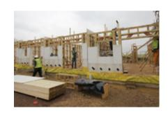
Another layer of 9mm Magply is also fixed across the inner face of the timber frame, followed by 25mm battens and plasterboard to create a service space and for the first time on this project we have also selected Magply – in conjunction with sub-contractor enviroREND – to be the render backing board for the exterior finish."
