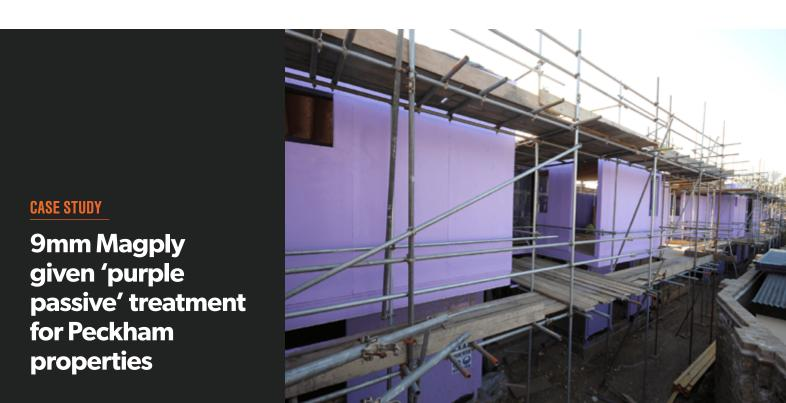
A development of two and three bedroom terraced homes on a brownfield site in South London is making use of Magply boards' fire resistance and other physical benefits: receiving a special polymer based, purple coloured membrane finish to provide excellent airtightness as part of an 'Eco-homes' energy specification.
