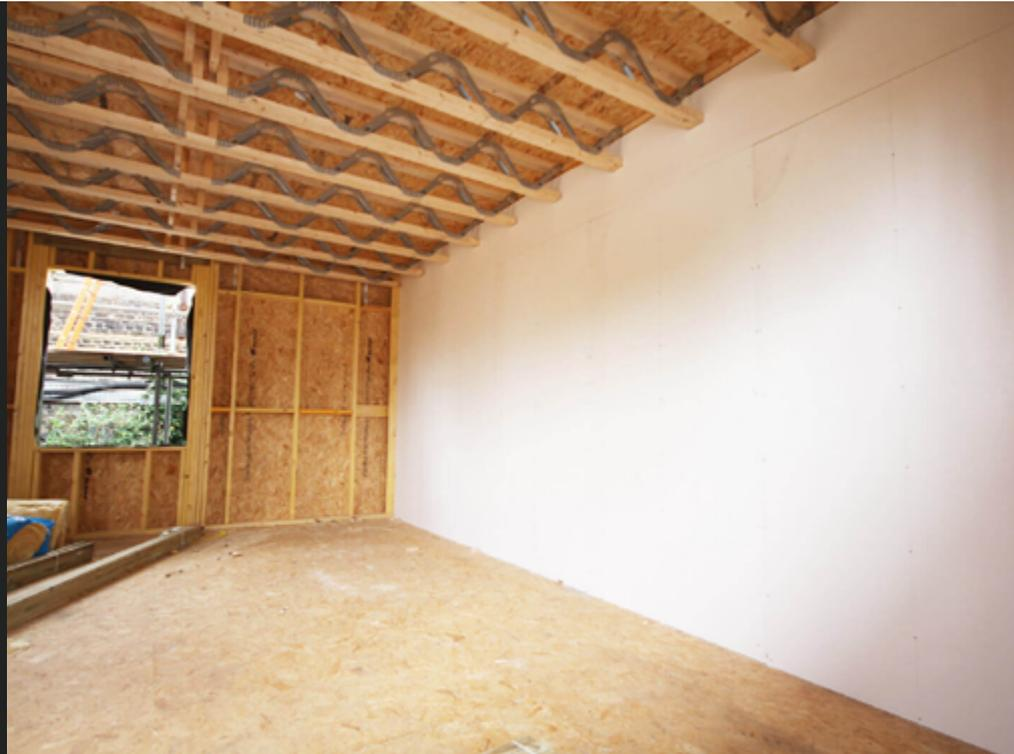
A 'shell & core' style apartment development in one of South London's up and coming districts is making use of Magply boards' fire resistance and other performance characteristics, as the lining to a bespoke timber frame package.
