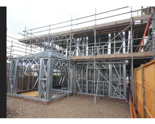
A cutting edge residential project in Essex is making use of Magply boards for both the internal lining and exterior cladding treatment to an innovative lightweight steel framing system, demonstrating the widely specified fire resistant product's multiple attributes.
