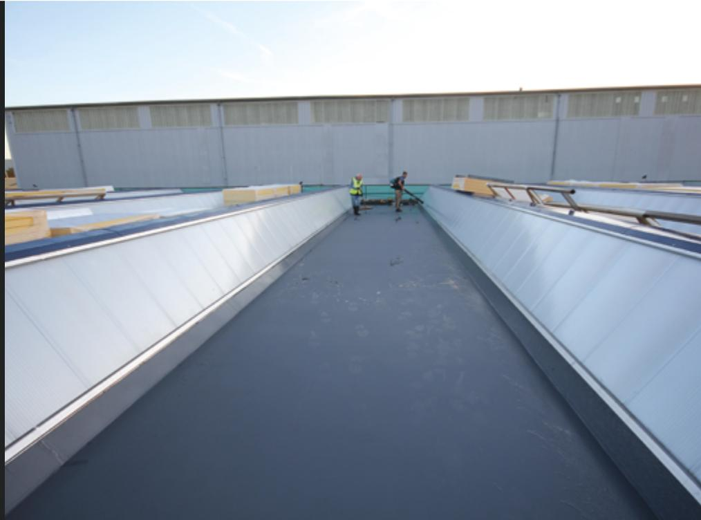
A Dutch manufacturer of fireproof flat roof coatings is recommending IPP Limited's Magply boards as the ideal substrate on which to install its liquid applied treatments: based not only on their fire rating and stability, but also because of the material's flatness.
